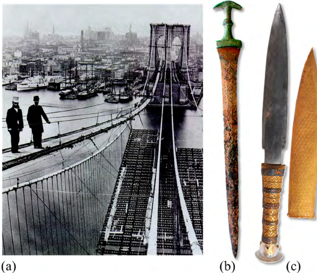
Figure 76. A few (extreme) examples of long-lasting iron products: (a) Brooklyn Bridge, built 1869–1883; (b) Hittite sword from the early iron age, about 1200 BC; (c) iron dagger of Pharaoh Tutankhamun, 1330 BC, manufactured not from reducing ores (because the Egyptian empire was in the bronze age at this time) but from an iron-nickel meteorite via forging. These examples show that time must be considered as an essential factor when estimating scrap return quantities.
